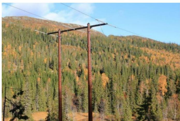
Figure 18-6 H-frame tension structure
