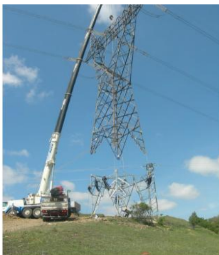
Figure 19 - Tower Lifting by Crane
