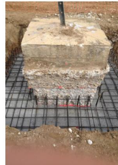
Figure 22 - Foundation trial pit and upgrading examples
