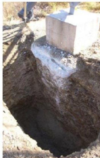
Figure 22 - Foundation trial pit and upgrading examples
