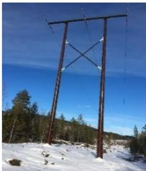
Figure 10-8 FRP cross-braced H-frame
