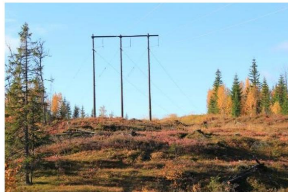
Figure 18-7 Angle tension structure
