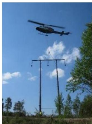
Figure 10-18 Placing a H-
