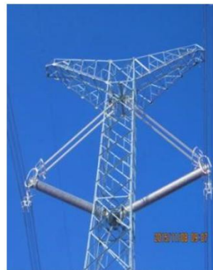
Figure 9-9 800kV DC hybrid tower, steel and FRP composite
