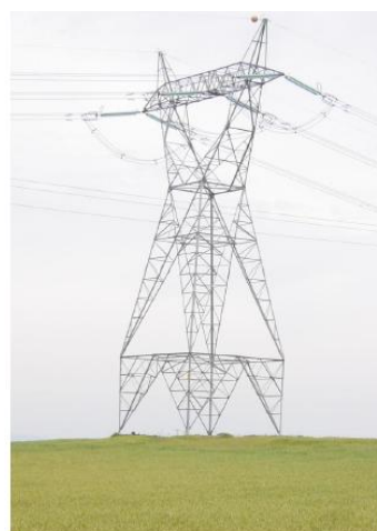
Figure 20 - Tower with bottom extension installed
